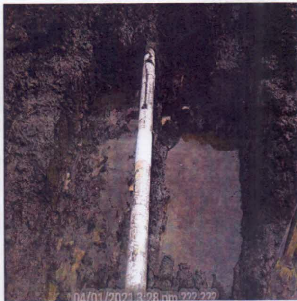
Fig D: Incident Facility after repair
